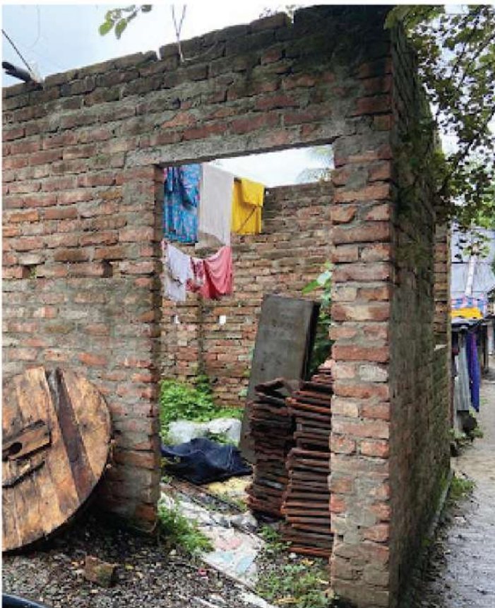
The school building of the slum before the intervention
